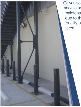
Galvanised steel bollards are an effective way to restrict access and highlight architecture and are virtually maintenance free. Offering an exceptionally long service life due to their durable galvanised steel material, these high quality bollards are a cost-effective way to protect any area.
